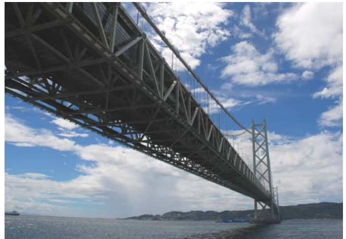
Figure 1.1. Akashi Kaikyo Bridge
