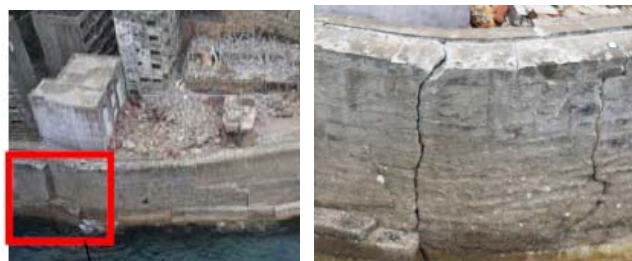
Fig. 5 The picture taken from the sky with a camera loaded onto UAV
